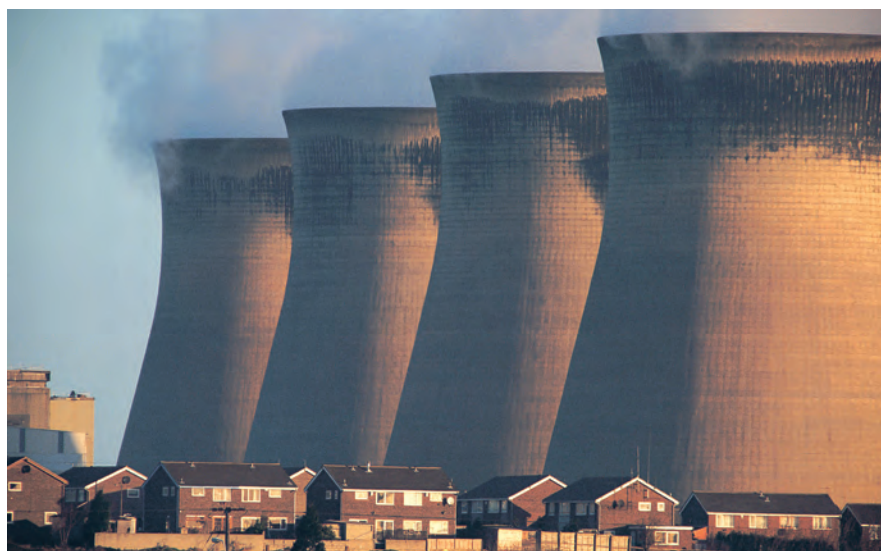
Cooling towers are a common sight near power stations. They are used to cool down the steam coming out of the turbine. This waste heat could be used to heat the houses nearby. This would increase the efficiency of the power station up to 70%.
